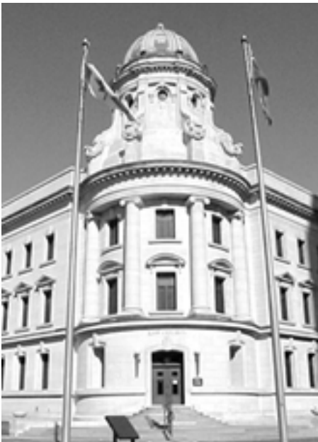
Historic Law Courts Building, Winnipeg
